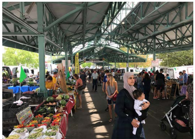
Open Air Pavilion at Overland Park Farmers Market (1990-2024) Credit: City of Overland Park
