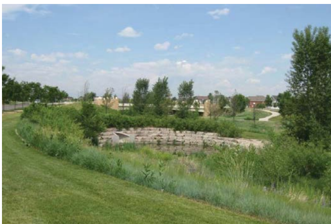
An example of a naturally designed drainage facility Credit: City of Denver
