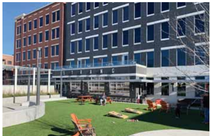
Strang Hall common consumption area, Downtown Overland Park, KS Credit: Rick Planning + Design
