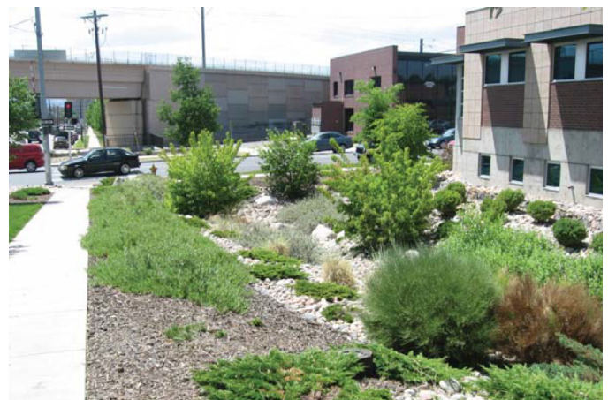
An example of a natural drainage facility with an adjacent multi-use trail Credit: City of Denver
