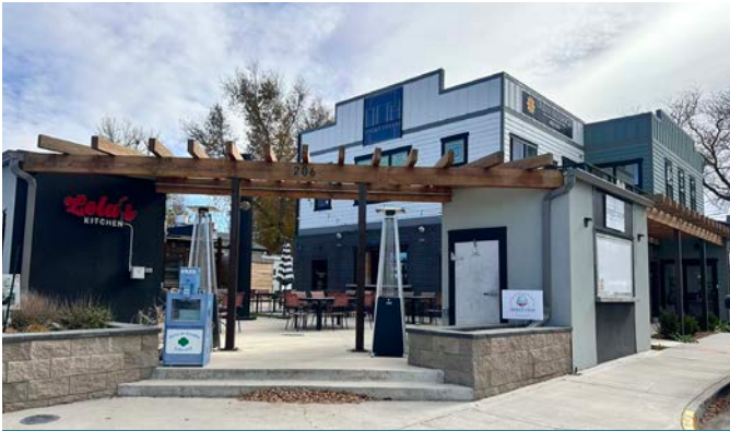
This newer building at Fifth and Elm Streets integrated the historic patterns of lap siding and windows common in Frederick during its peak as a mining town. Credit: RICK
