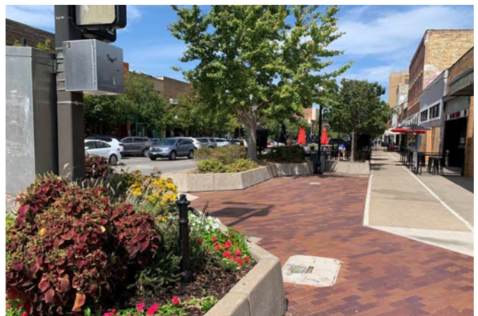
Bulbout with landscaping at a downtown intersection Credit: RICK
