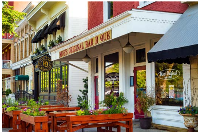
Example of a building front incorporating glass, kick plates, large picture windows, varying exterior surfaces, and a recessed entry Credit: Shutterstock
