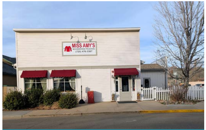
This newer building, at Fifth and Elm Streets, used horizontal lap siding and vertically oriented windows to mesh with the historic architecture patterns in Downtown Frederick. Credit: Town of Frederick
