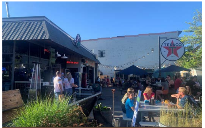
Conversion of a Texaco gas station to a pizza and brewpub in Downtown Durango, CO Credit: RICK
