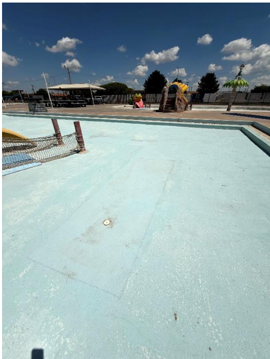
Ship Pool – Inlet Repair
