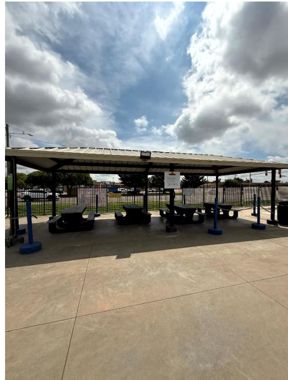
Metal Shade Structure
