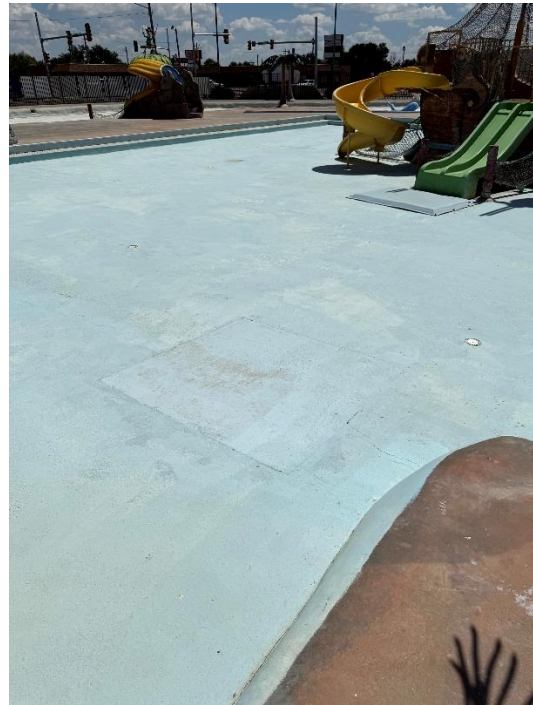
Ship Pool – Patch Repair
