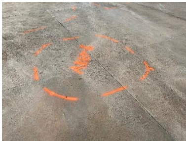
Photo 11 shows Area 8 from west to east.
