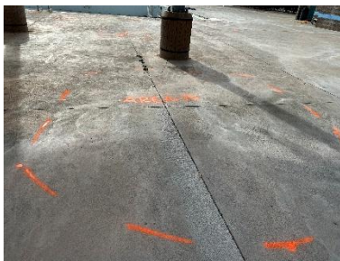
Photo 13 shows Area 10 from north to south.
