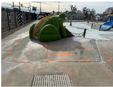
Photo 8 shows Area 4 from north to south.
