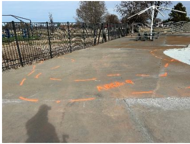
Photo 12 shows Area 9 from south to north.
