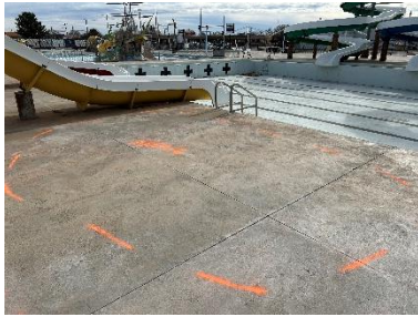
Photo 9 shows area 6 from northwest to southeast.
