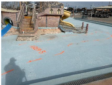
Photo 8 shows Area 5 from south to north.
