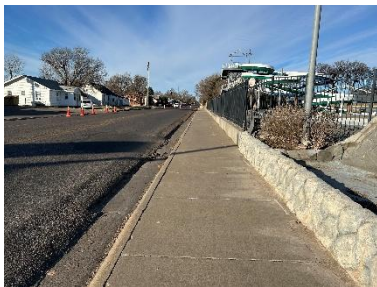
Photo 6 shows the sidewalk to the south from east to west.
