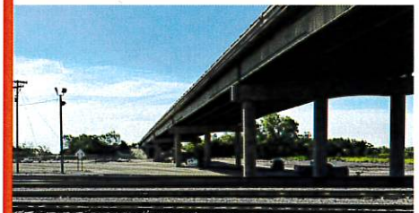
US-50 over BNSF Railroad Railyard
