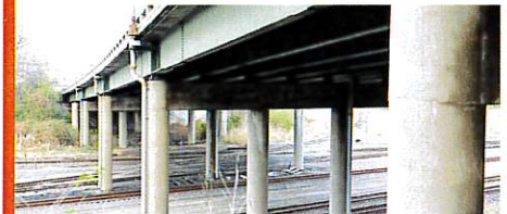
Central Avenue over UP Railroad Railyard
